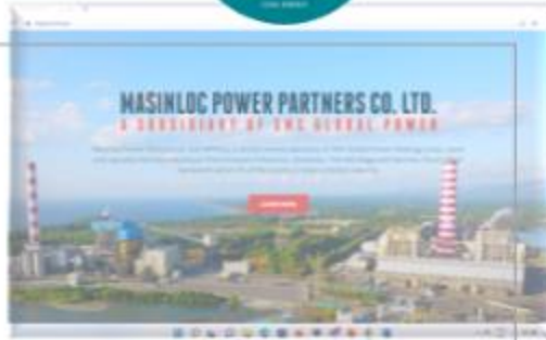
Masinloc Power Partners Co., Ltd, Zambales
